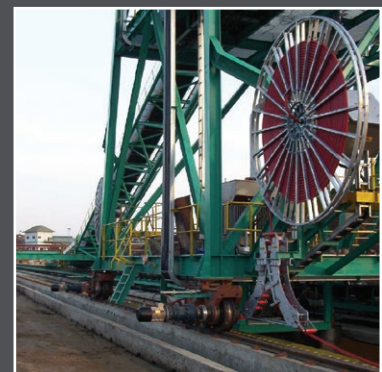
Motor Driven Cable Reel on a Stacker/Reclaimer, Thailand, Travel Length: 380 m
