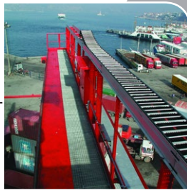
Energy guiding chains for the main trolleys on automated RMGs
